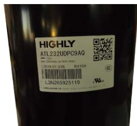
Compresor inverter R410A HIGHLY ATL232UDPC9AQ
